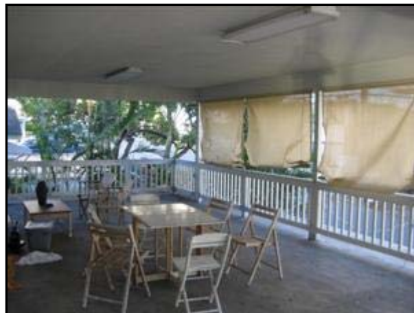
2.0 Picture 7 Upper Level Front Deck
