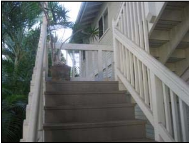
2.0 Picture 5 Exterior Stairs
